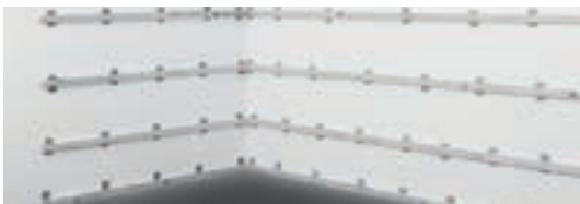
Timber battens straight onto wall
